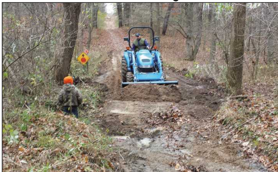
VOLUNTEERS WORK to repair a trail in Allegan County in preparation for the upcoming snowmobile season.
