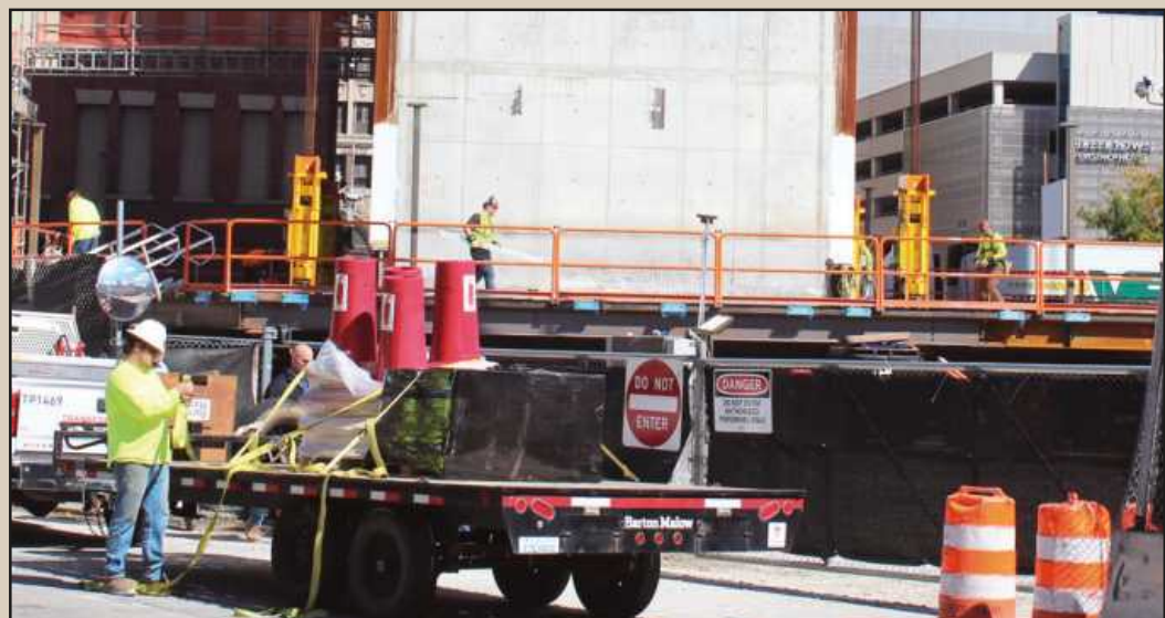
TYING MATERIALS to a trailer leaving the Exchange Building site is Shane Sheridan of Laborers Local 1191. He's employed by Barton Malow. Behind him tradespeople are working on the 10th floor of the building, which will be raised and locked into place.
