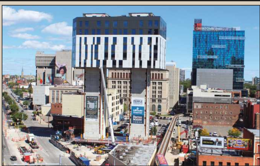
THE EXCHANGE BUILDING in Detroit is being erected unlike any other structure so far in North America – from the top down. Doing the work to erect the 16-story building on the edge of Greektown are project manager Barton Malow/LiftBuild, its subcontractors and building trades union members. At this point in construction, from last month, the 11th story is the most recent floor that has been lifted into place.
